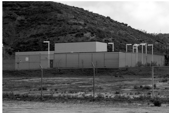
Sewage boost pump
